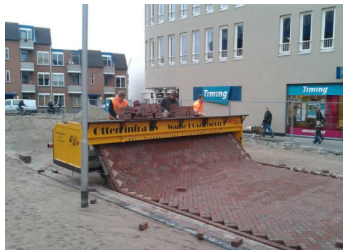
How brick streets are laid in The Netherlands
